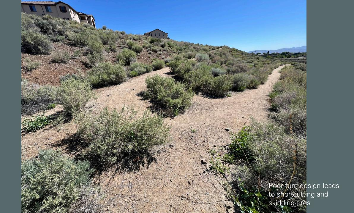
Turn Profiles Poor Design - erosion prone Sustainable design – soil stays in place
